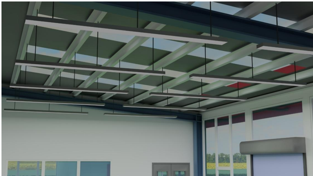
Figure 119 – Lighting lamps in the workshop
